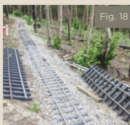
Fig. 18: Track panels ready for installation near mile-post 8-2 on the low line.
