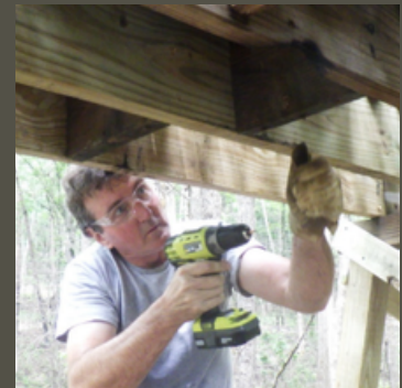
Fig 5: Dale installing one of the blocks between stringers to help keep them spaced properly. The Kimball trestle was done by mid-June and the focus shifted to completing the Hobbstown trestle.
