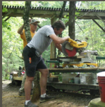
Fig. 4: Dale King cuts a length of 2" x 6" while Barry Garard observes. Barry and Dale did a lot of the stringer and bent work on this trestle. Many others helped here as well.
